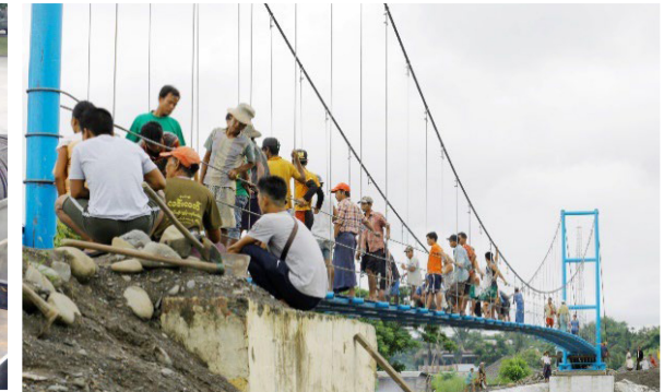
Pedestrian bridge in Myanmar built with cables from donated second-hand cables SOURCE: Corentin Fivet, Jan Brütting, Nothing is lost, nothing is created, everything is reused: structural design for a circular economy, The Structural Engineer, vol. 98(1), p. 74-81, 2020
