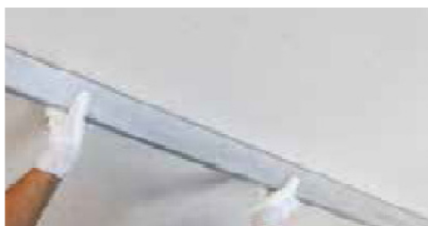
Figure 38 — Façade planarity check
