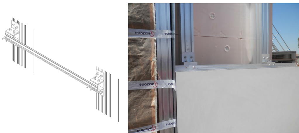
Figure 53 — Placement of supporting horizontal profiles
