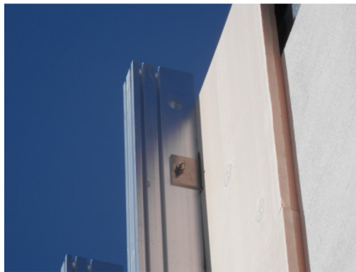
Figure 43 — Upper fixation already placed
