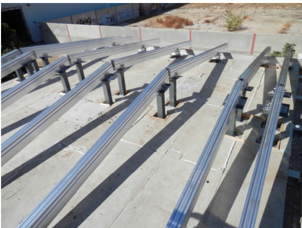
Figure 58 — Placement of secondary substructure
