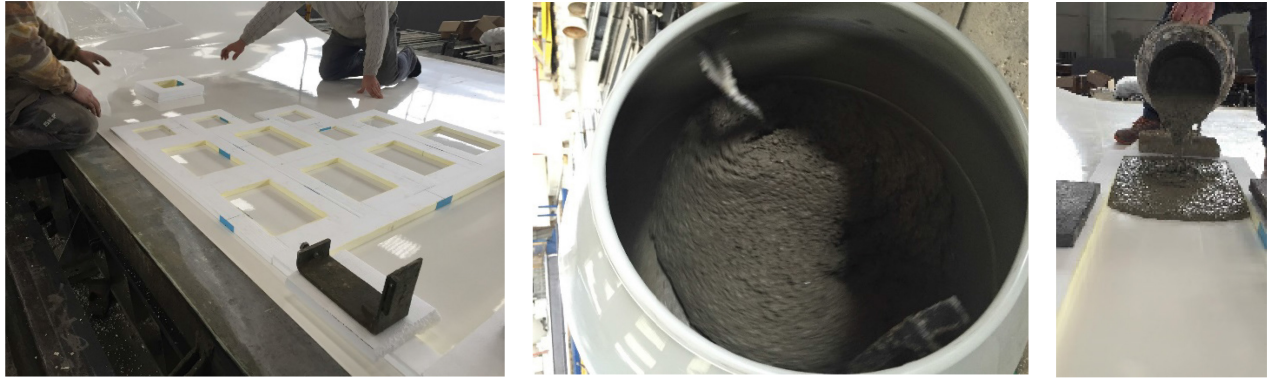
Figure 19 — Preparation of the formworks, Mixing of the concrete and Concrete casting in the formwork
