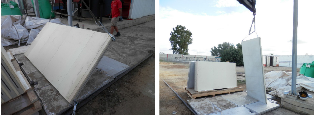
Figure 25 — On-site storage and lifting of Multifunctional Insulated Panels
