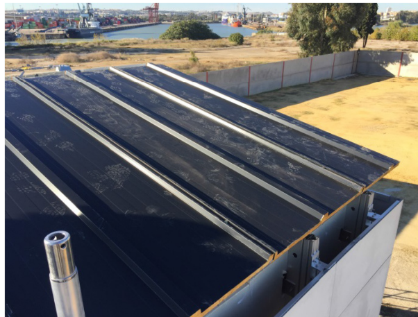
Figure 61 — Placement of sandwich panels
