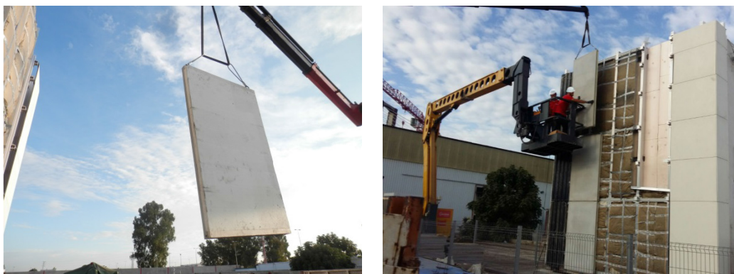
Figure 49 — Placement of Multifunctional Insulated panels in real case
