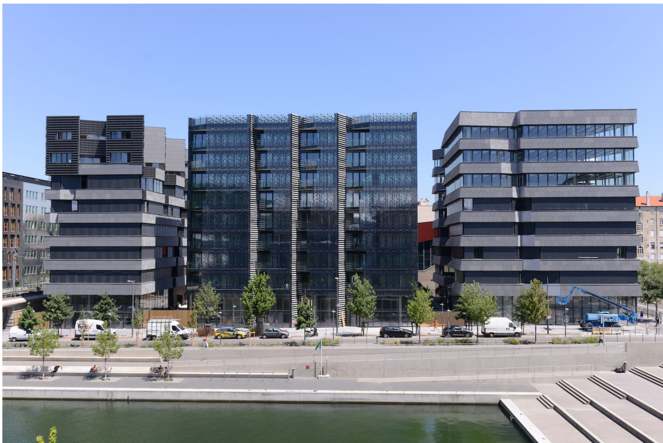
Figure A.1 — HIKARI, a 12.300 m 2 positive energy block located in the Lyon-Confluence area designed by Kengo Kuma (architect) and Bouygues Immobilier (real estate developer) with a 190 kWp PV system [4]
